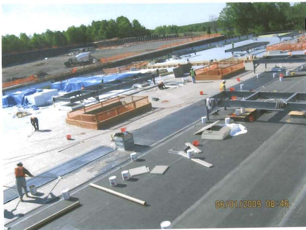
Unit #2 Roof Area (6/1/09)
