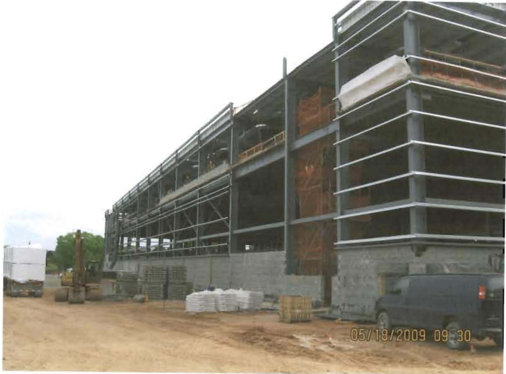
Overview of the Building area viewed from South West Corner (5/18/09)
