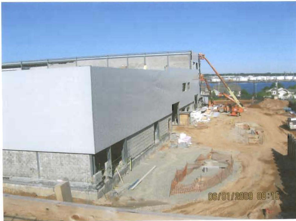
Overview of the Building area viewed from North East Corner (6/1/09)
