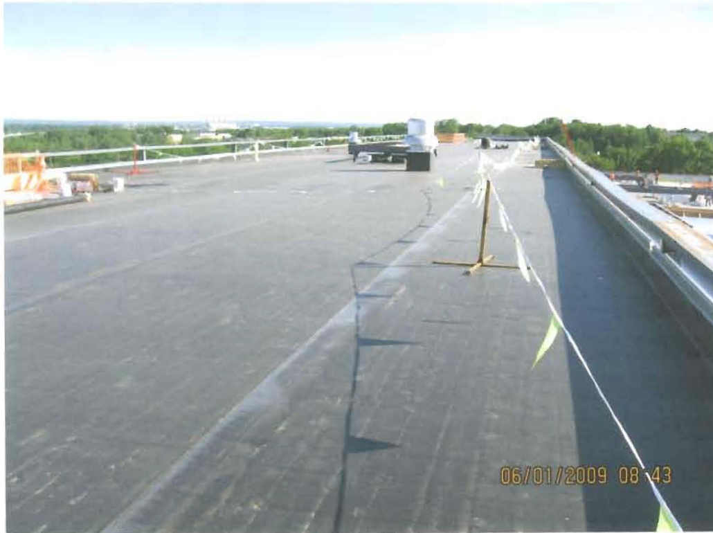
Unit #1 Roof Area (6/1/09)
