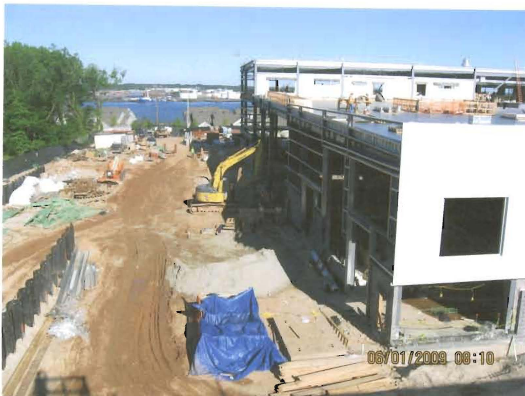
Overview of the Building area viewed from South East Corner (6/1/09)
