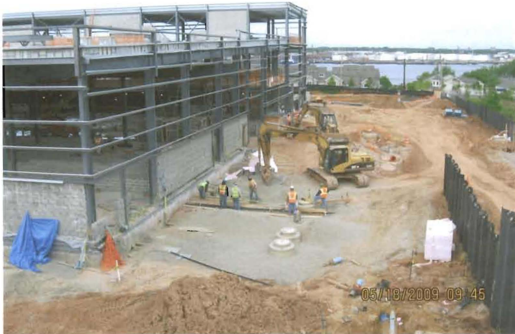
Overview of the Building area viewed from North East Corner (5/18/09)
