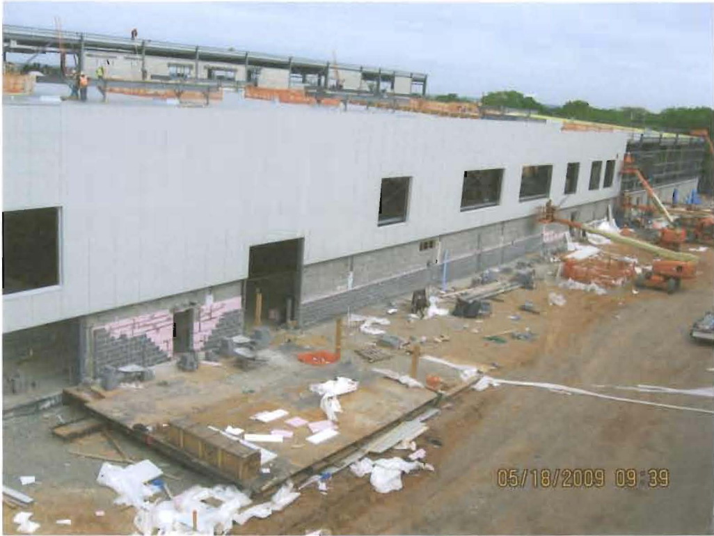
Overview of the Building area viewed from South East Corner (5/18/09)
