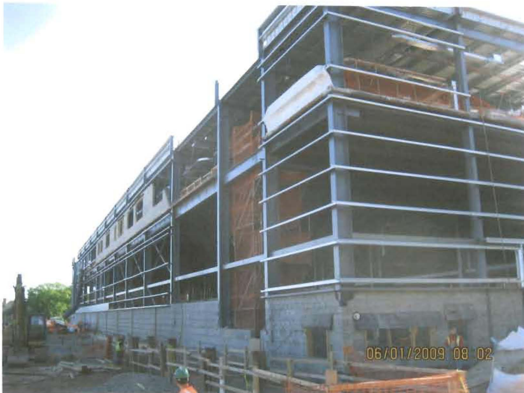
Overview of the Building area viewed from South West Corner (6/1/09)
